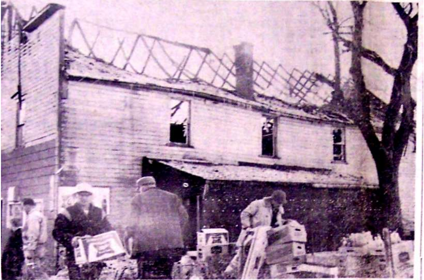
Several hours after the fire that destroyed the Cushing Tavern Saturday was brought under control, volunteers were still moving equipment and stock away from the scene. Here the volunteers are carrying merchandise to the Ed Olson building just north of Goldsworth's Cushing Tavern. The sixty-four-year old building was so badly damaged by fire, it was declared a total loss. Action of the new Sterling Township fire department was credited from preventing possible further loss.
